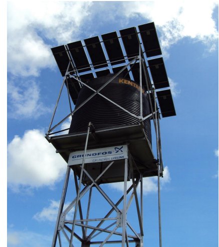
Figure 1- Katitika LIFELINK tank and solar panel
